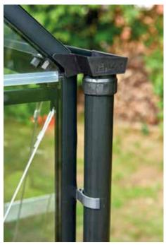
**Downpipe**Downpipe for rainwater collection
