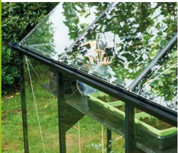
**The glass is fitted using glazing capping**, ensuring a beautiful finish. The capping is a neat alternative to clips, which damage the overall aesthetics and allows dirt to accumulate around them.
